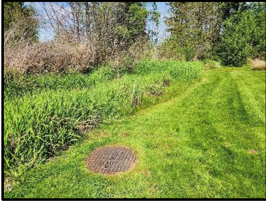
Detail of sewer manhole at wetland edge
