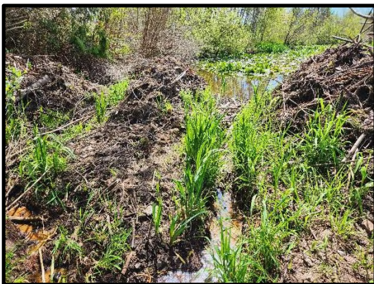
Detail of dam outlet
