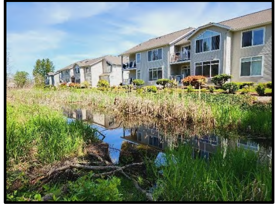
Wetland proximity to houses south of the south pond
