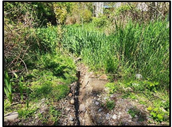
Secondary outlet at the NW edge
