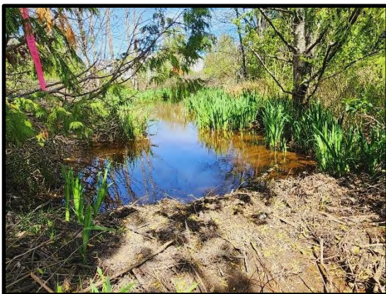
Additional dam between ponds
